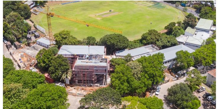
New School of Education under construction
