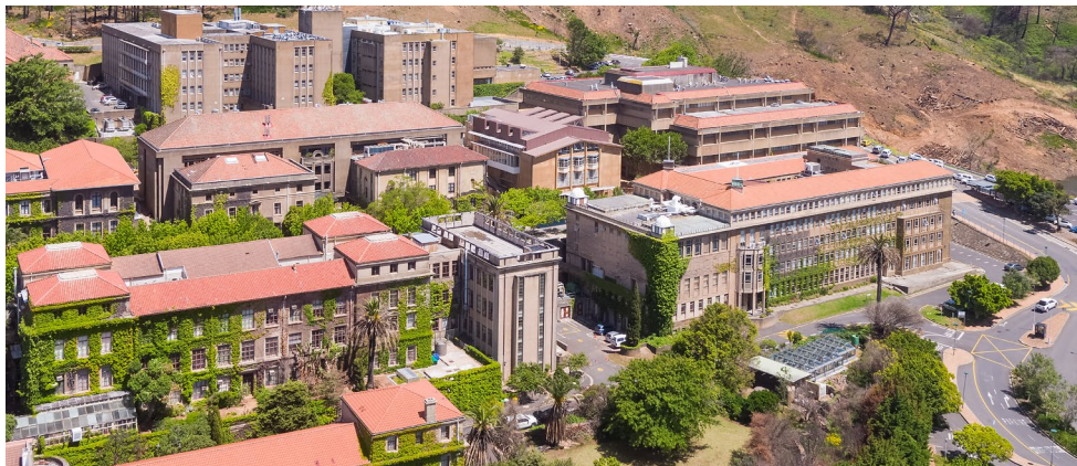
Aerial view of Upper campus with fire damage repairs in process
