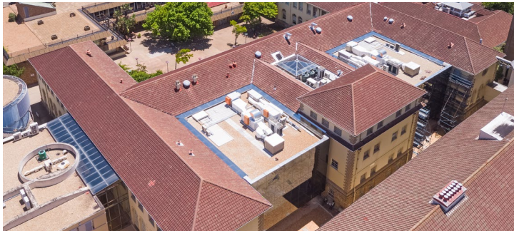
Aerial view of UCT IDM Infill extensions
